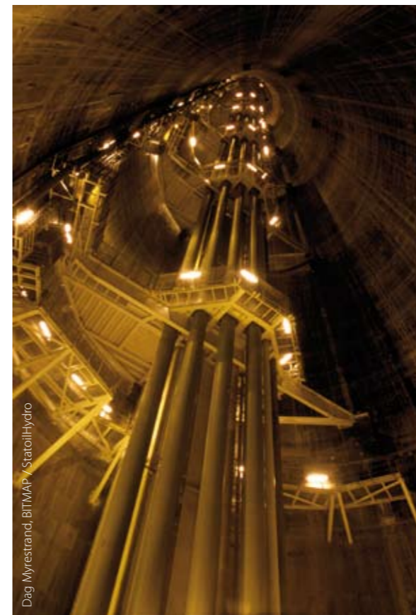
The concrete shaft of the Statfjord A platform extends 330m (1083 feet) below sea level.
